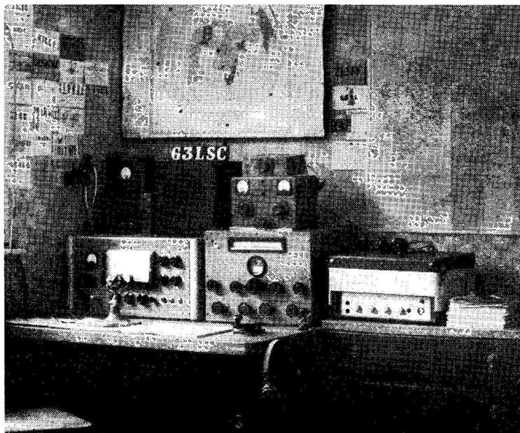
G3LSC is at Poole, Dorset, and started with the Top Band Talking Box — see "Short Wave Magazine," October 1956 — and a CR-100 receiver. Though he still has the Talking Box, the main transmitter is now a K.W. Vanguard, with a Cubical Quad for the 21 mc band. For 160 metres, he has a 250ft. wire, so arranged that the middle 30ft. section is in the vertical — another approach to the problem of getting the current antinode, where the radiation occurs, into the right place.
