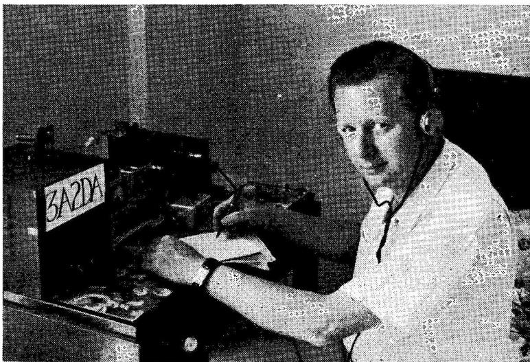
3A2DA (G3CWL of Leatherhead) was on the air during June 18-22, with 10 watts to a 5763 and an ARC5/R26, modified for one-band operation on 20 metres, as receiver. With a dipole on the roof of the hotel, some 50 contacts were made in a total operating time of about 15 hours. The gear, specially contrived for the trip, was part of the luggage in a vintage Austin Seven.
