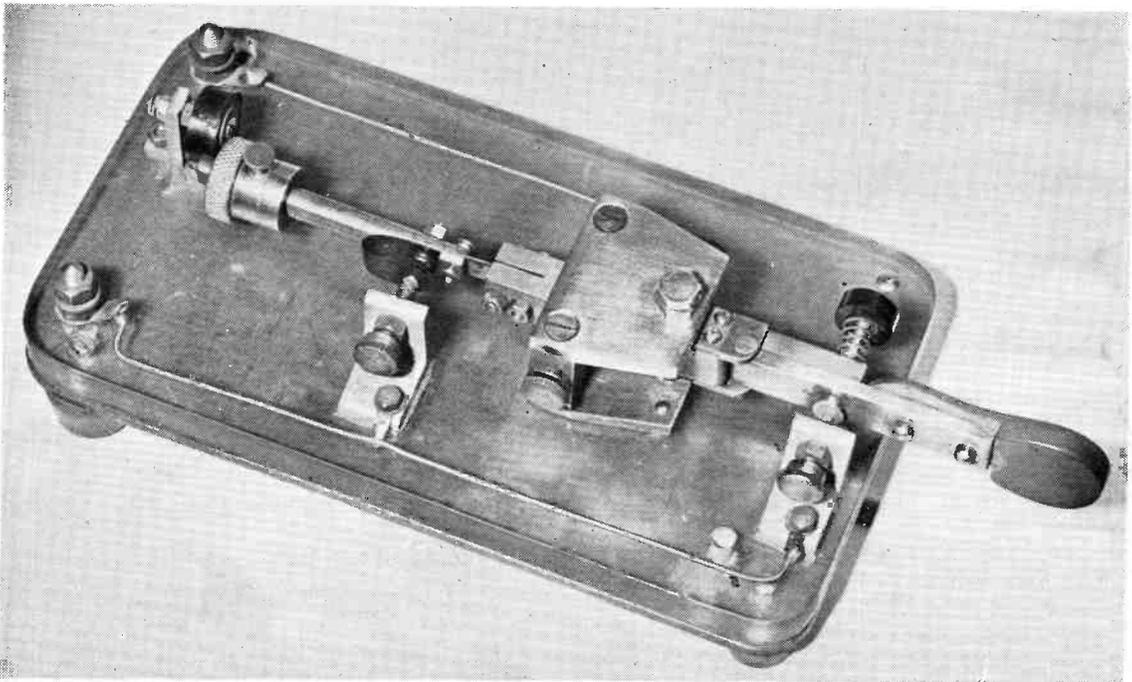
The neat finished appearance of the semi-automatic Morse key made by G3BIK and described in his article. The action on such a key is quite different from that of the straight or "pump-handle" variety; once it has been acquired, the average operator can send better Morse for longer periods than is usually possible on a straight key. The operation of a semi-automatic key is very definitely something that must be learnt with an audio oscillator on closed circuit, and not over the air!
