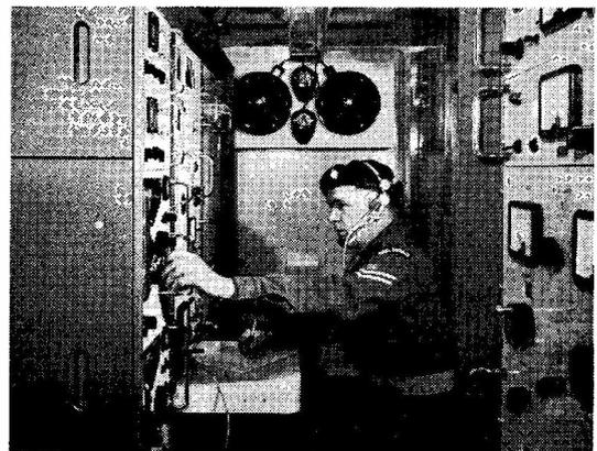
Inside the signals office of the Racal HF transportable station, with the receivers and control console at left, and the transmitter unit at right.
