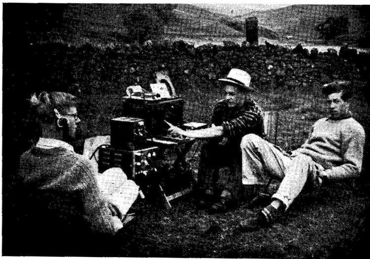
The GM3NVO/P outfit when G3NVO (hat), G3NVN (right), G3NVV (phones) and G3OHX (who took the photograph) were in Roxburgh working GDX on Top Band. In four evenings, some 60 contacts were made, the aerial being a 300-ft. wire, with a kite-borne quarter-wave vertical flown when possible.
