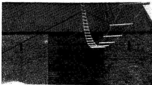
A view of the 600-ohm open-wire feeder, at 3-in. separation on plastic spreaders as described in the text, in position. The lateral lines about half-way along are nylon cords, loosely secured to convenient supports, to prevent too much movement under windy conditions. The set-up as shown here has easily survived severe gales from all directions. (In this photograph, the continuation of the feeder above the roof is “lost” against the sky.)
