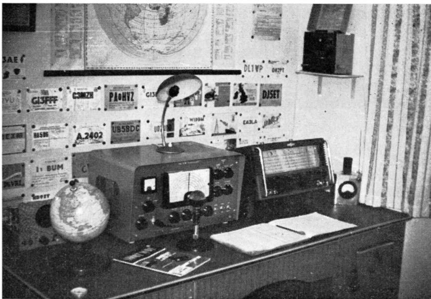
THE station of GI3IEO—owned and operated by W. B. Johnston, 146 Ulsterville Park, Portadown, Northern Ireland—has been developed over a period of almost exactly ten years, to that shown here. The ticket came through in March 1952, and a start was made with QRP CW on 160-80m., using a 6V6 in the PA. After various other transmitters home-built to SHORT WAVE MAGAZINE designs (all of which worked very well), the first commercial venture was with a Panda "Cub" Tx and an Eddystone S.640 receiver.
