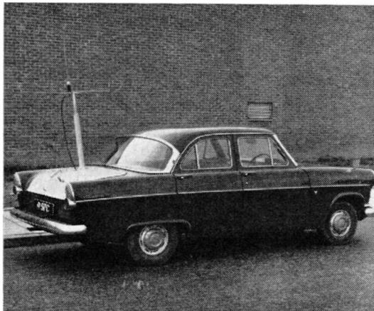
The retractable position for the Clark telescopic aerial mast, as fitted to a Ford Consul. The handle for pumping up the mast can be seen on the lid of the boot — see text for notes on the design and application. Extended view overleaf.
