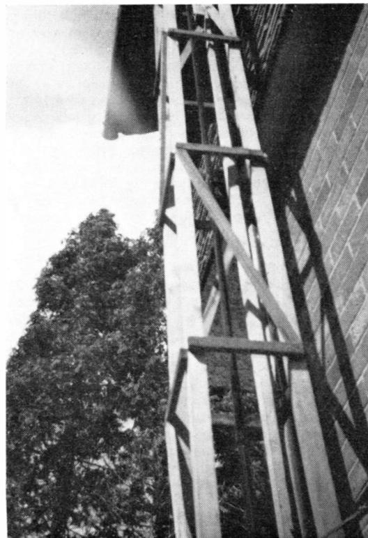
Close-up of a section of the mast described in the article — and see drawings which, when read with this view, make the fabrication clear. The central element is the metal tube (actually 1-in. electrical conduit) for driving the beam head, and the coax feed-line is also run up this tubing — see text.
