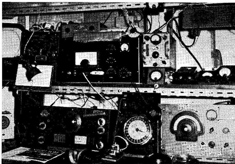
Operated by G3FYE and G3PEK, the Stockport Radio Society signed G6UQ (which is the Club call sign) for the recent MCC, and came up in second place with 554 points. Their Tx is a Panda Cub, the receiver an HRO, and the aerial a half-wave. G6UQ is installed at the Stockport Radio Society headquarters.
