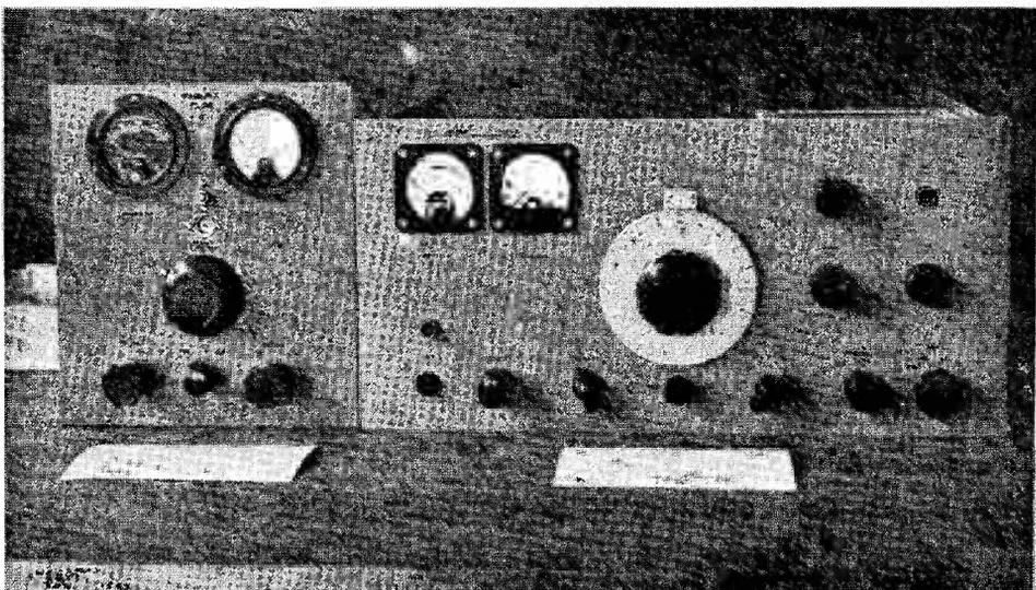
This was one of the home-constructed items in the Cornish Radio & Television Club's exhibition at Penzance on June 15. Built by G3OCB of Truro, it is a 10-160m. SSB exciter giving 40w. p.e.p. with, at left, a two-metre PA operated on the transverter principle, through an oscillator-mixer unit.
