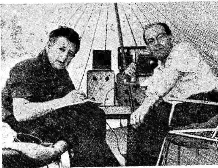
The operating position, PX10X, Andorra, with DL2AG on the microphone and SWL Brian Balchin logging. The gear, fitted up in their living-tent, consisted of a K.W. Viceroy and a Drake 2B receiver. Except for some trouble due to power supply variation, which caused a 500-cycle drift on the Tx, it all performed faultlessly. The band mainly used was 20 metres, in the SSB mode. In a total operating time of 49 hours, 720 contacts were made in 64 countries and 171 of the QSO's were with U.K. stations.
