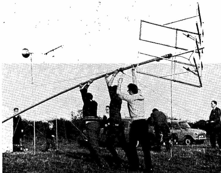
Raising the 70 cm. aerial when the Bristol group turned out for a recent VHF field-day. Working the 23 cm., 70 cm. and two-metre bands, they raised eight stations and heard ten more, on 70 cm., with G3LTF as best GDX logged; G2CIW was also heard. The two-metre 6-ele Yagi and 23 cm. bowl reflector are shown in the background.
