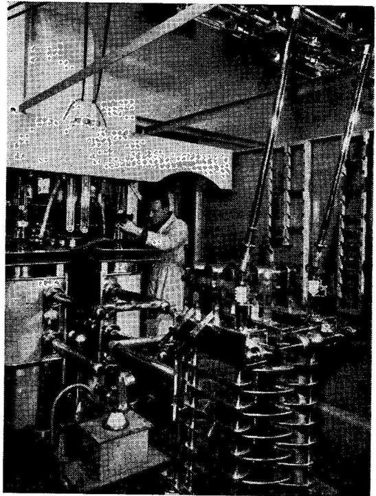
You may be running what in Amateur Radio would be called QRO — but look at this for a tank circuit! The output end of the RF power amplifier on one of the 100 kW HF transmitters for Radio Australia, at Shepparton, Victoria.
