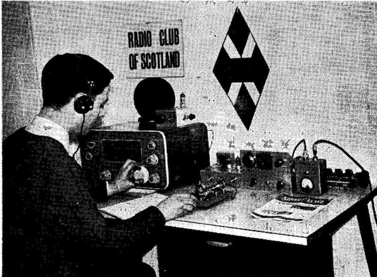
Neat Top Band rig at GM3RCS, of the Radio Club of Scotland. The station was specially assembled for the 1964 MCC; the operators were GM3LTB, GM3SAN (seen here) and GM3SJU. Their Tx was to a "Short Wave Magazine" design, using a 6BW6 in the PA, and full BK with a valve-type T/R switch. The receiver was a Minimitter MR44/II, and the aerial an inverted-Vee with a maximum height of 38 feet. In 16th place, and leading the Scottish entry, GM3RCS made 492 points.
