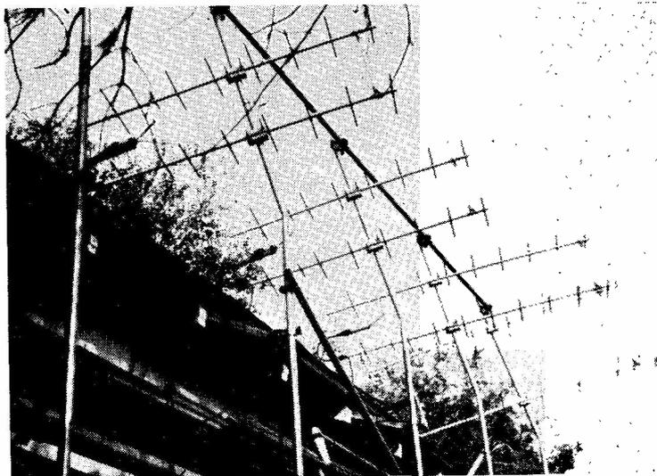
You would hardly believe it, but this collection of VHF arrays, at the home station of W6YY, is part of his multi-channel set-up for the remote control of his real DX station at the top of Mount Wilson, twelve miles away and nearly 6,000ft. up! About 30 different control channels are available. They certainly do things in a big way out in California!
