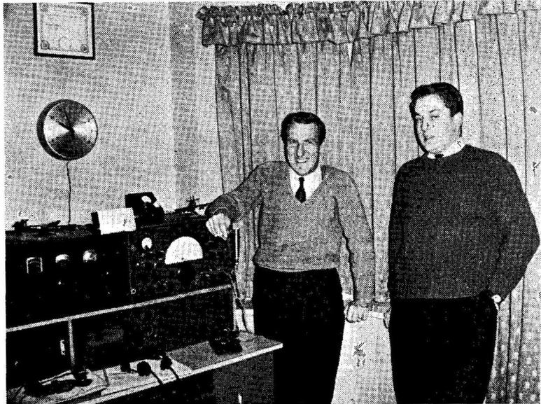
Running G3SRC of the Surrey Radio Contact Club (Croydon) into ninth place, tied with Harwell No. 2 (G3HS) — on the left, G3BFP, with G3MCX. Their transmitter was the 160m. section of an all-band SSB rig, the receiver an AR88D, and the aerial a loaded 160ft. wire. The station is that of G3BFP. *A G6LX print*
