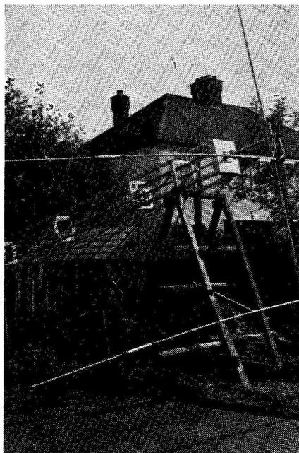
(B) A seven-foot high support cradle, or "launching pad," was made for the G3SM 40-foot tower, here seen ready to go up with the TA-33Jr. beam in position.
