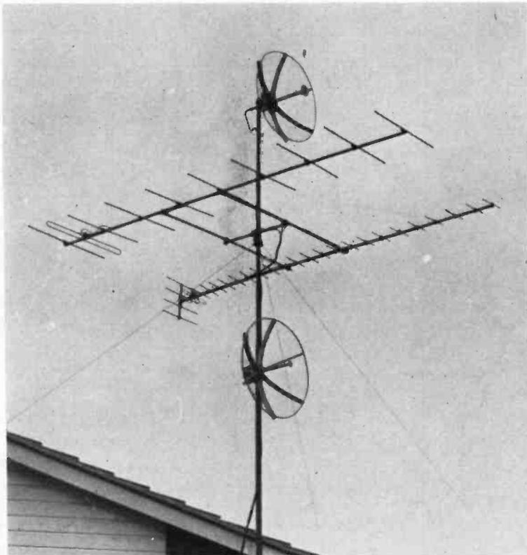
(Above) the VHF/UHF aerial system in use at G3ZEZ, 16 Kestrel Way, Clacton-on-Sea, Essex. At top is a 3 ft. dish for 23 centimetres—then a 10-ele Yagi for two metres—below it a 24-ele array for Seventycems—and lastly a 3ft. dish for 3 centimetres. Mounted on a rotatable mast, the whole of this assembly is home-built. At lower left is the station of G3ZEZ, all the VHF gear having been constructed by him. Altogether, a very workmanlike job, on which he is to be congratulated.
