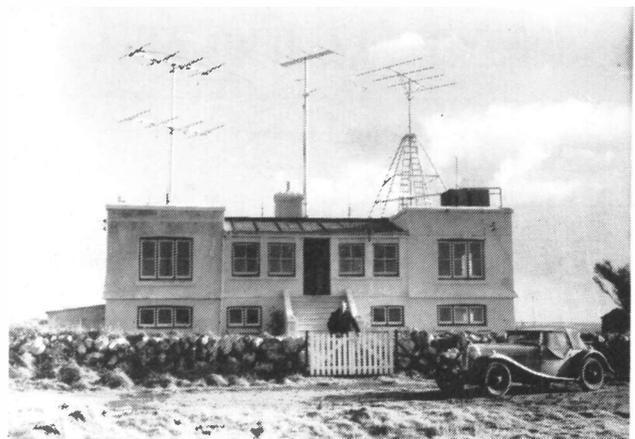
General view of the VHF beam installation at G5BY, Bolt Jail, South Devon, in December 1947. On the left, two wide-spaced 4-ele 58 MHz beams; a close-spaced 51 MHz 4-ele is at the centre with, on the right, an all-metal wide-spaced 50 MHz beam.
