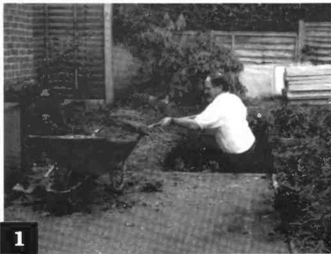
Apart from the mast and rotator cage, you will need a fine weekend, 0.5m<sup>3</sup> of  $\frac{3}{4}$  in ballast, two bags of cement and some muscle-power. The ground post requires a concrete base 1 x 1 x 0.5m, so get digging! Keep an eye open for any drains, underground cables or pipes and position the centre of the hole far enough away from your boundary to keep the antenna from overhanging your neighbour's property and well clear of overhead lines.
