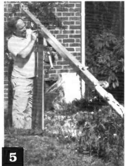
**5** This is the bit that really needs an assistant (he had nipped off to take the picture). The main mast is lifted onto the ground post and the pivot bolt inserted. The instructions suggest that a temporary support is used to hold the top of the mast level while you are doing this. In my case the ground sloped upwards so I didn't bother. The assistant will probably need to move the mast around to allow the bolt to slip in easily.
