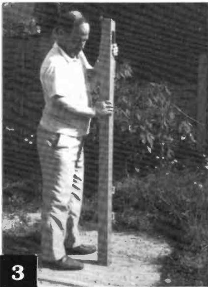
**3** The ground post plugs into the socket - provided that you have kept it clear of concrete. Don't be too impatient - the concrete needs several days to harden. Beware of frost in winter and protect the new concrete with a thick layer of sacking. In summer cover it with a polythene sheet to prevent it drying out too quickly. Before inserting the ground post into the socket smear thick grease all over the part of the post that will be in the socket.
