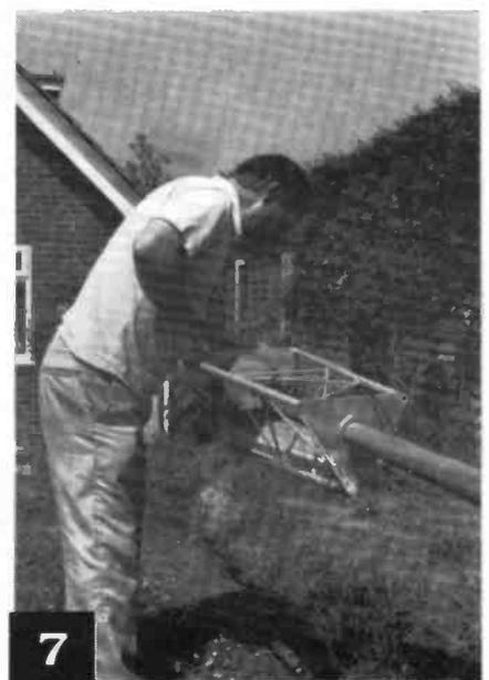
**7** The rotator is housed in a galvanised steel cage which clamps onto the top of the upper section of the mast. Tennamast can supply cages drilled to suit any of the popular rotators. I used the rotator which had seen eight years service at the top of my pole. If you are using your old rotator then I recommend that you service it before bolting it in place - I didn't and the main bearings had disintegrated!
