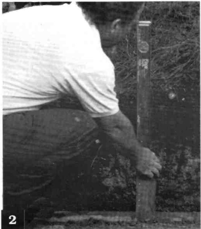
Unless you want your mast to emulate the Leaning Tower of Pisa the ground socket must be vertical in all directions. Check with a good builder's spirit level, wedge the socket with bits of rubble and recheck. When filling the hole with concrete put a polythene cover over the open end to keep the tube clear of concrete. Don't forget to keep checking that it is vertical and carefully tamp the concrete to ensure that it is properly compacted.
