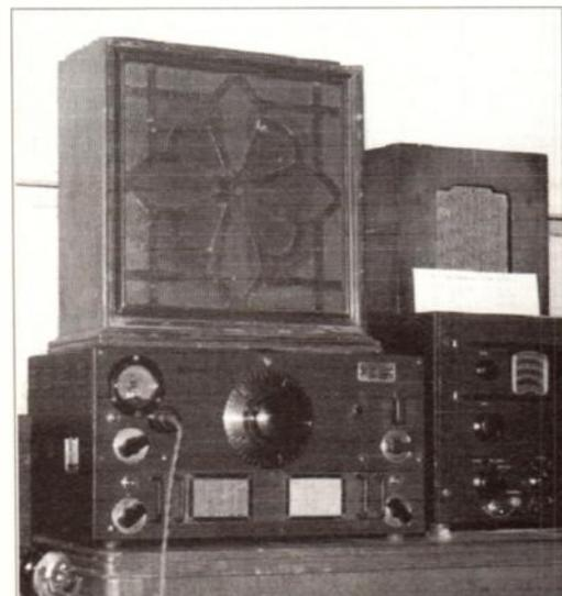
**Two types of communication receiver used to receive the coded signals that were fed into Colossus.**
