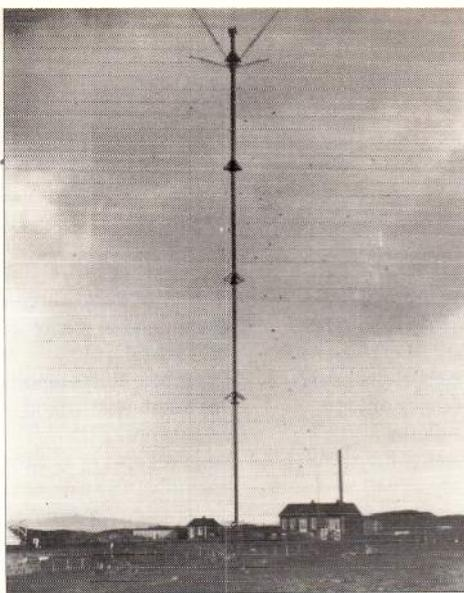
**Machrihanish 122m tower and station showing the 'Umbrella Capacity' shrouds, insulated guywires, and ball and socket base.**
