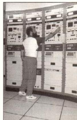
Although the transmitters can be completely controlled by computer, the technicians must be prepared to manually select the on/off time, frequency, appropriate antenna, antenna take-off angle, antenna slew angle and programme. Each of the ten 500kW transmitters has a control rack. Four of the racks are shown here.
