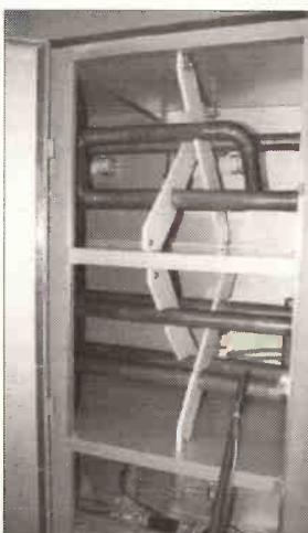
Shown here is one section of the anode inductor for the transmitter. Large diameter copper pipe is necessary because of the high power levels involved.
