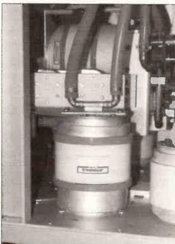
Vacuum capacitors used in the transmitters are water-cooled. There's no shaft to turn the rotor plates here!
