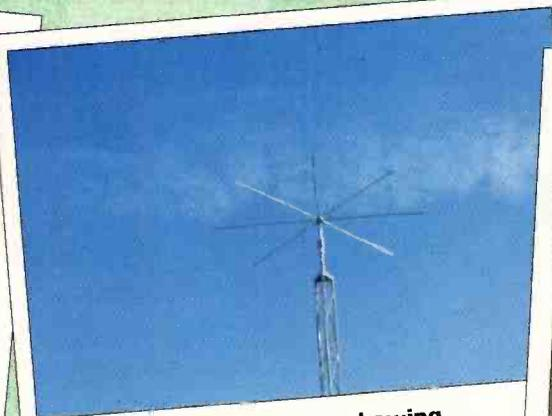
Top of Monopole Antenna showing capacity hat and loading coil.
