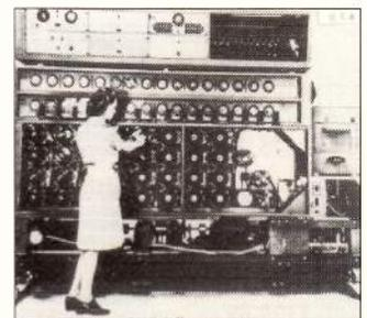
American 4-rotor Bombe (front view) being operated by a 'WAVES'.
