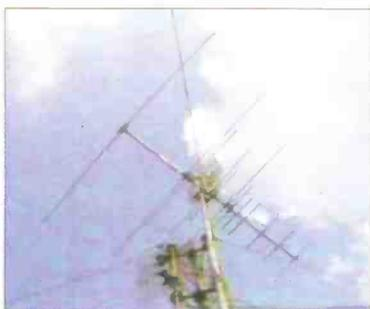
A typical lattice mast installation used for DXTV reception.
