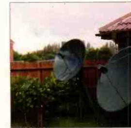
The home teleport, the 1.2m distant dish uses a Chaparral dual band LNB some seven years old with ferrite polariser (and OK for digital!) but shortly a lower noise (0.5dB) Gardiner LNB and mechanical polariser will be fitted. The nearer dish is a 1.5m for C-band, both dishes are green to minimise visual impact and neighbour anguish.
