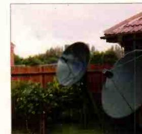
The home teleport, the 1.2m distant dish uses a Chaparral dual band LNB some seven years old with ferrite polariser (and OK for digital!) but shortly a lower noise (0.5dB) Gardiner LNB and mechanical polariser will be fitted. The nearer dish is a 1.5m for C-band, both dishes are green to minimise visual impact and neighbour anguish.
