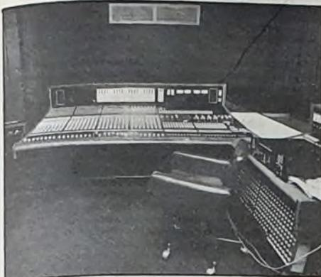
Control room featuring 32 input/16 output desk with 24 track monitoring and advanced correction facilities
