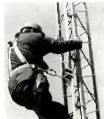
The IBA's Safety Officer, fastened to a transmitting mast by means of a special harness, tests safety procedures adopted by maintenance staff.
