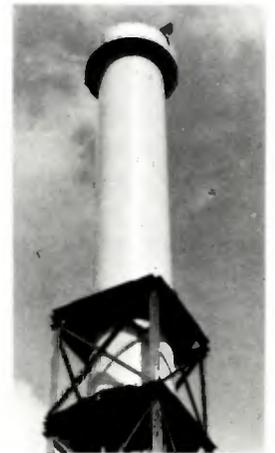
A 3ft diameter cylinder containing UHF transmitting aerials mounted in a special cradle to allow tests to be carried out near the ground. Later the complete unit will be taken to the transmitting station and lifted and fixed many hundreds of feet above ground. (EMI)
