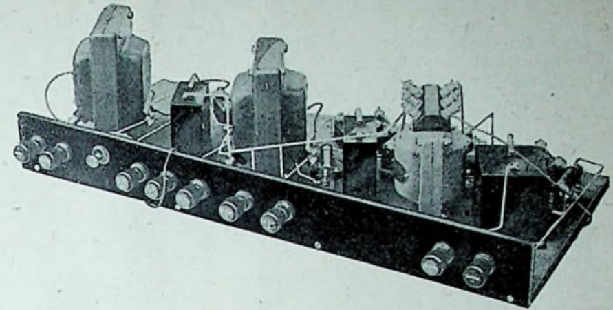
Another view of the amplifier showing more clearly the angle at which the L.F. transformers are set.
