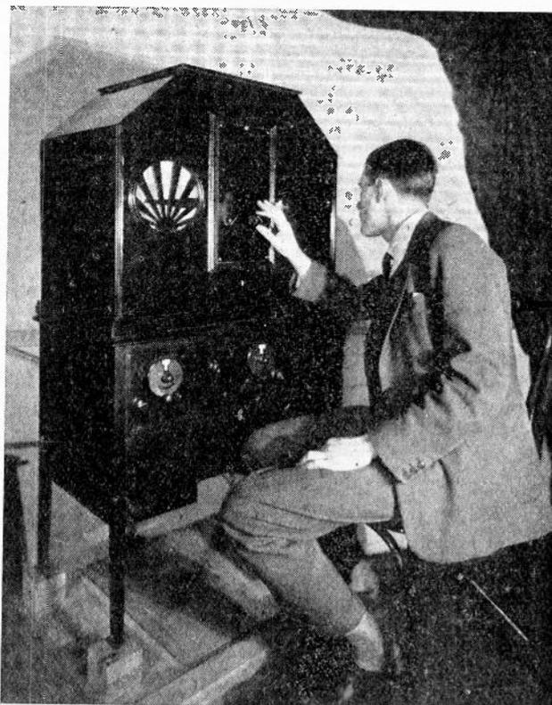
*Receiving a Television transmission on a Baird Dual Exhibition Receiver. The apparatus shown contains two wireless receiving sets, one for speech and one for vision. The "televisor" is fitted with a Baird automatic synchronising apparatus.*
