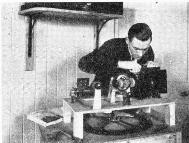
Busy with the construction of a Baird "Televisor" from a kit of branded parts.
