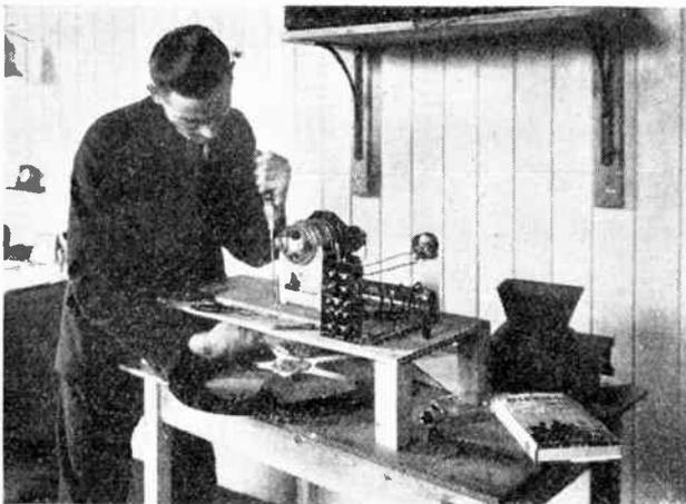
Busy with the early stages in the construction of a Baird "Televisor" from a kit of parts.
