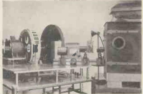
Fig. 3. A photograph of the double-image polariscope employed in conjunction with the Wilson scanning system.
