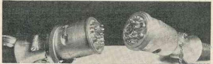
*Special junction unit for connecting multi-core cable between the cameras and the control equipment. The cable used is capable of passing a frequency band of 3 megacycles without appreciable distortion.*
