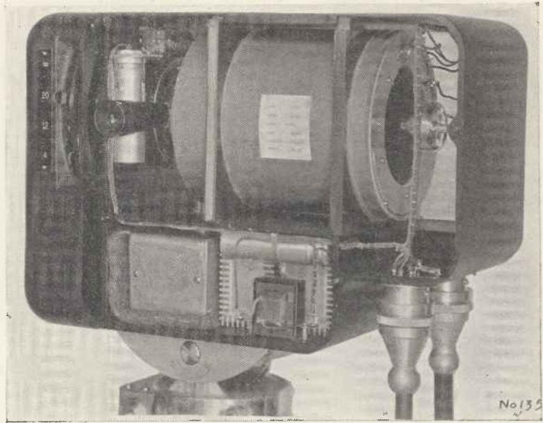
*A photograph of the new Farnsworth television camera with one side removed showing the construction.*
