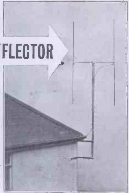
Illustration shows a "Belling-Lee" Mast-Head Television aerial with reflector. The aerial is a simple centred half-wave Dipole consisting of two weather-proofed tubings of correct proportions to give maximum reception of the vision channel at 45 M.C.
