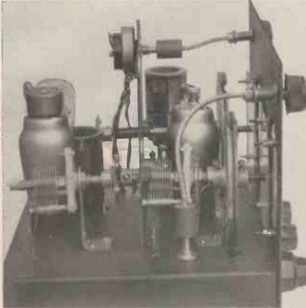
This is the opposite end of the receiver showing the flexible coupler going to VC6 which tunes to wave trap circuit.
