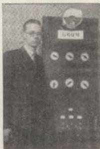
This station of G6QM is operated off D.C. mains with a rotary converter.
