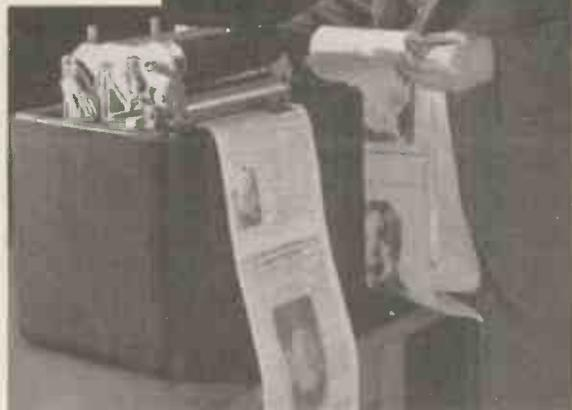
the facsimile material is printed is 8½ in. The length of each page is 12 in. on a continuous roll. Printing speed is at the rate of three feet of record per hour. A time clock arrangement at the printer-receiver automatically turns the apparatus on and off in accordance with a pre-determined transmission schedule.
