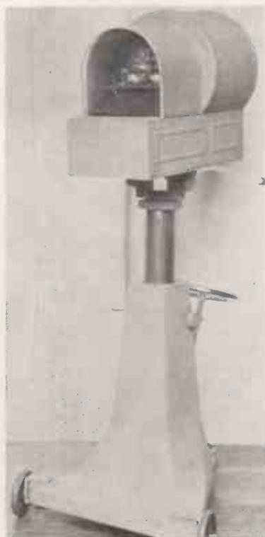
Fig. 5. (Left) Iconoscope camera for studio use.
