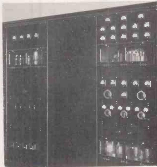
This is the transmitter at W9XUP which is now operating on 26.150 Kc. and relaying the N.B.C. red network programmes. The power input to the final is 1,000 watts.
