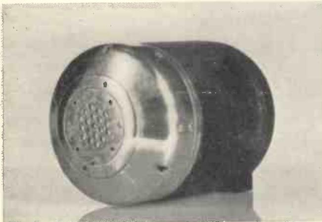
Fig. 4. Moving-coil microphone used at Alexandra Palace.
