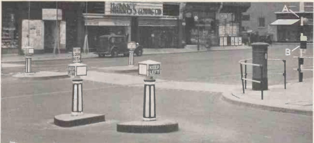
Pedestrian crossing, with Bollard illumination controls. A contains the light-cell and B the control gear.
