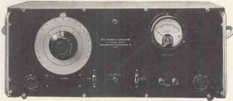
A Marconi-Ekco mains-operated oscillator of the heterodyne type covering the audio frequency range between 10 and 12,000 cycles per second. The harmonic content is low and the output voltage is sensibly level over the whole frequency range.
