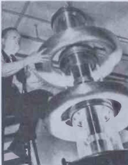
Fig. 7. Construction of individual glass X-ray tube sections.
