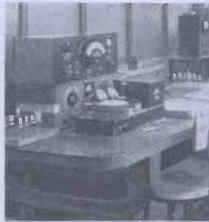
Fig. 6. At this bench the finishing work necessary to adjust the performance of the crystals to meet specified requirements is carried out.
