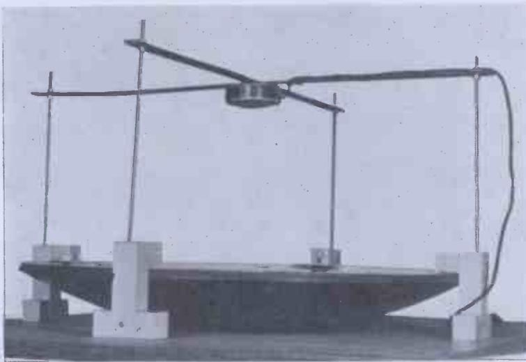
Photograph showing means employed for positioning microphone at focal point of reflector.
