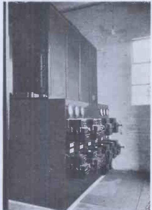
Installed in March 1929 at Victoria & Exchange Station Manchester, these Westinghouse Metal Rectifiers have been in constant use ever since operating D.C. point machines direct from an A.C. supply.
