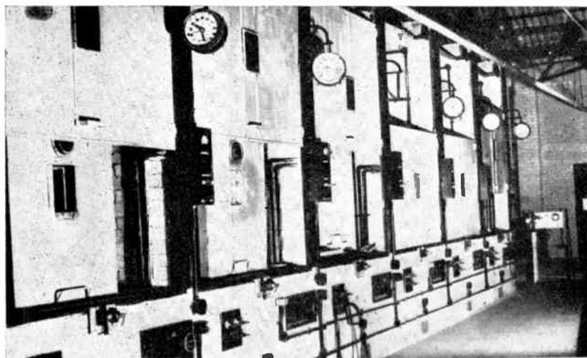
Fig. 5. Exhaust units for tubes operating up to 220 kV.
