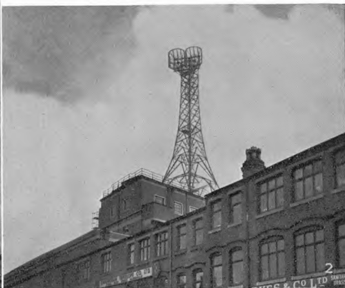
Fig. 1.—Exterior view of Dunstable repeater station, showing aerial arrays erected on a temporary mast. The buildings at the foot of the tower house the standby generator, equipment, the transmitter-receiver, power and monitoring equipment.
