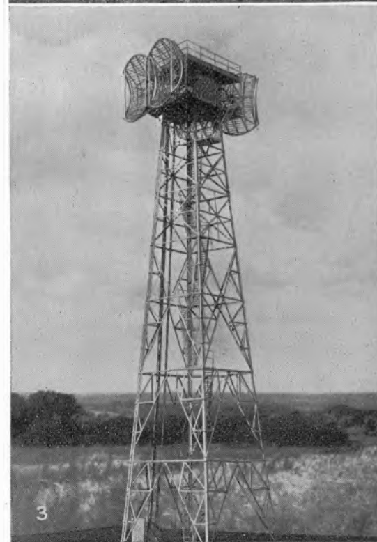
Fig. 1.—Exterior view of Dunstable repeater station, showing aerial arrays erected on a temporary mast. The buildings at the foot of the tower house the standby generator, equipment, the transmitter-receiver, power and monitoring equipment.
