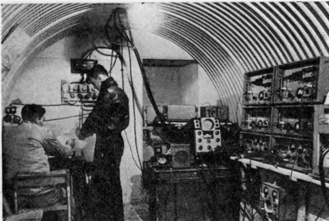
The repeater station near Calais which occupies a German dugout in the Cap Gris Nez area. The photograph shows the two sets of portable units.
