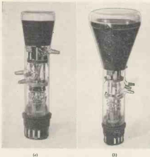
Fig. 1(a). G.E.C. cathode-ray tube type 908BCC. (b) G.E.C. type 1608BCCA with post deflexion acceleration
