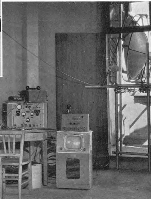
(below): Television transmitting equipment in the Hotel de Ville, Calais, together with monitoring and V.H.F. communication equipment. The transmitting microwave paraboloid can be seen on the extreme right of the photo.
