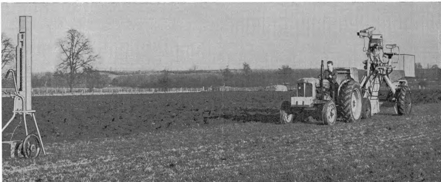
The gradient controller in use for drain laying
