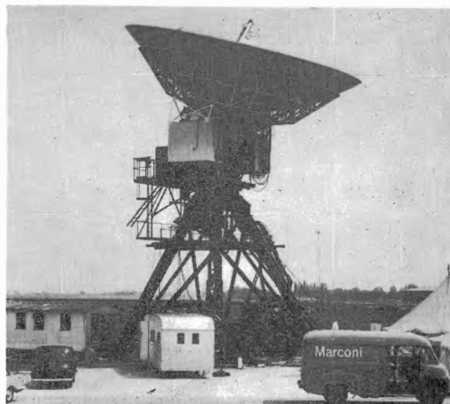
The 42ft parabolic dish aerial and its associated transmitting and receiving equipment mounted on a temporary tripod during the construction and testing at Rivenhall.
