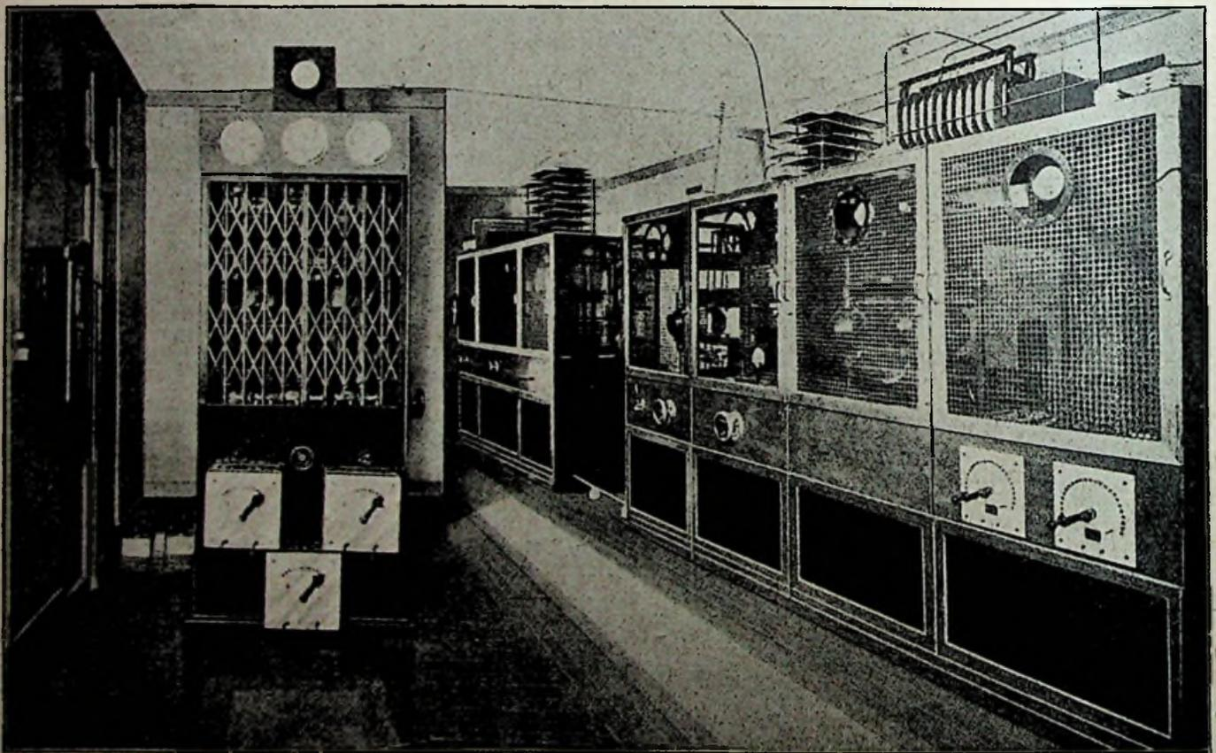
The arrangement of the transmitter at Radio-Toulouse, which has an output power of 8 kw., and broadcasts on a wavelength of 390 metres. This is one of seven French stations which, we learn, have decided to broadcast the Baird system of television.
