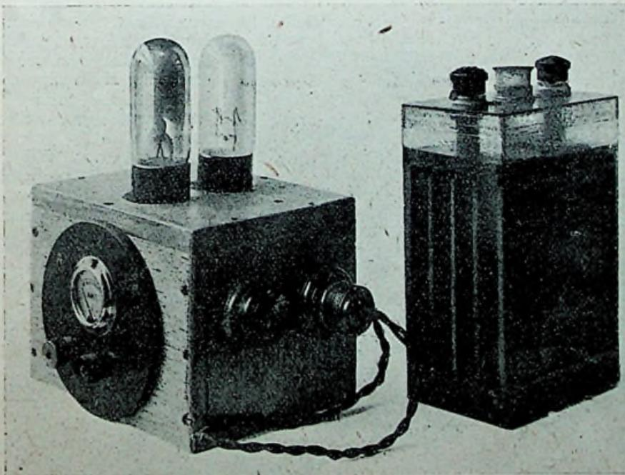
The rectifier with 2-volt 20 amp.-hour accumulator beside it. The buretter is the clear valve at the back. There are also shown the plug connection to the mains, switch, and output terminals with ammeter above them.
