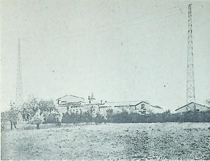
An exterior view of Radio-Toulouse, showing the masts and aerial. The station is situated three kilometres from Toulouse, on the plateau of Balma, which is 180 feet above the surrounding plain. The aerial is 180 feet long and 100 feet high.
