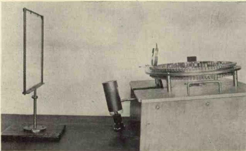
A general view of the Mihaly stationary mirror drum. In the receiver with which the demonstration was given an ordinary projection lamp was used, the light being modulated in a Kerr cell.
