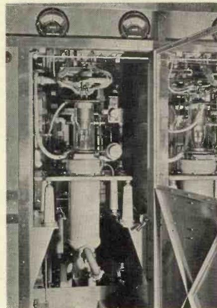
*Vital point in the Droitwich giant's transmitting equipment—one of the mighty valves in what the engineers call a C unit.*
