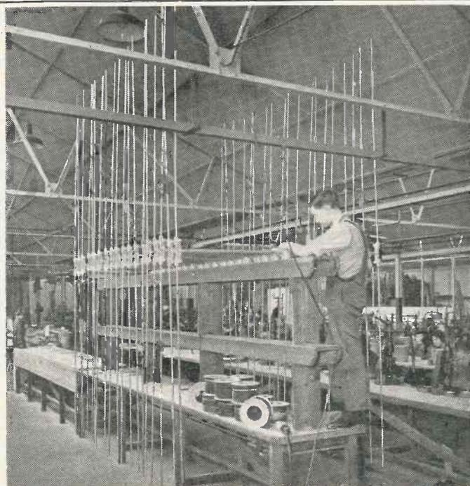
A batch of dipole aerials in course of construction at the Belling Lee works
