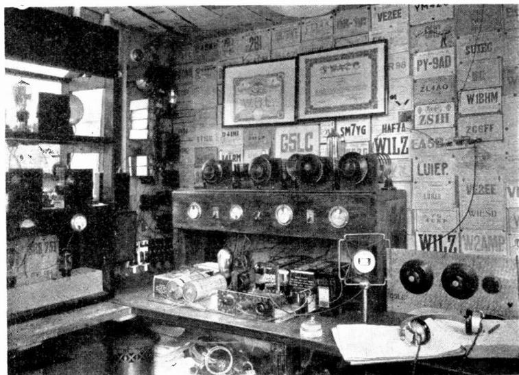
G5LC has worked all continents with this transmitter. Series modulation is used while the P.A. runs at 50 watts C.W. and 12 watts for phone. It is licensed for all amateur bands.
