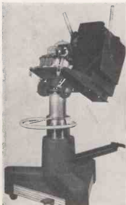
Left : Model KE2B2 studio camera equipment, rear view. Camera case open.
