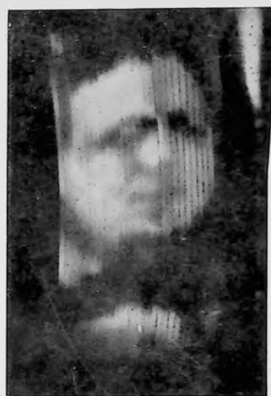
The first photograph of a television image ever published, the image on the screen of Mr. Baird's first televisor in 1926
