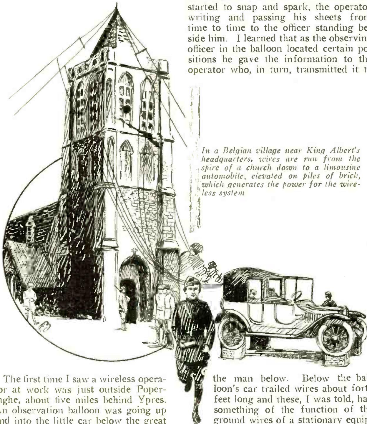
*In a Belgian village near King Albert's headquarters, wires are run from the spire of a church down to a limousine automobile, elevated on piles of brick, which generates the power for the wireless system*
