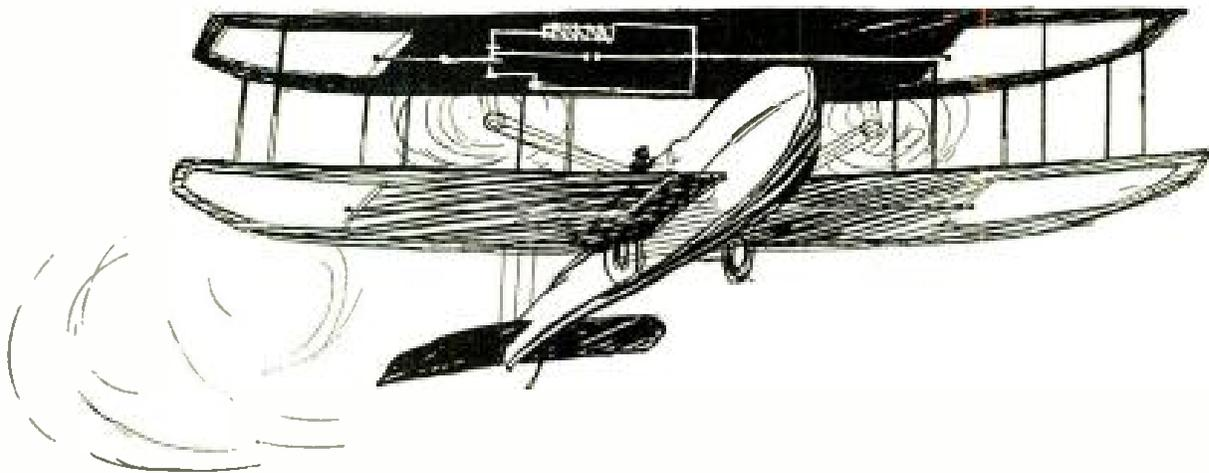
*Fig. 10.—Wireless-equipped aeroplane without antenna. The inventor has substituted two extended surfaces of conducting material, so as to form the two capacities of a horizontal antenna. From these surfaces, made of aluminum foil, conductors are run to the signaling instruments*
