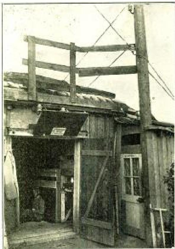
*Electric power station in the trenches. These stations are often used for transmitting power to the wireless installations*
