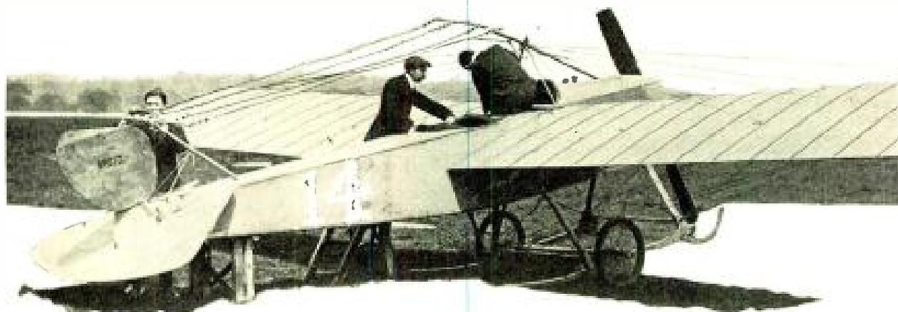
*The successful wireless experiments by aeroplane carried out at Hendon. Mr. Valentine's Bristol monoplane is being fitted with the installation, only 40 feet of wire being necessary to complete the station on the aeroplane. The experiments proved successful*
